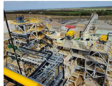
**Fig. 1:** Feed classification circuit wet commissioning
