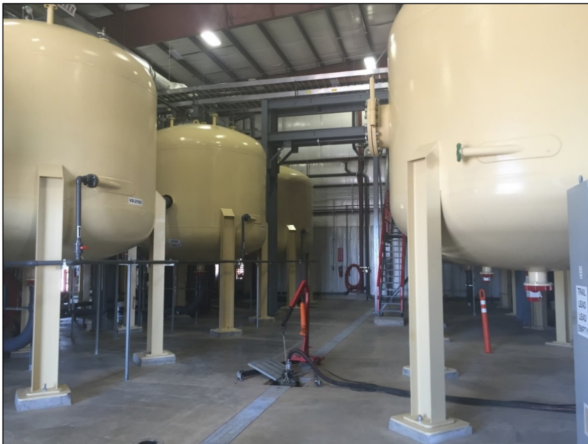
Figure 4-35: Ion exchange resin beds at Lance Project as of 1 June 2016
