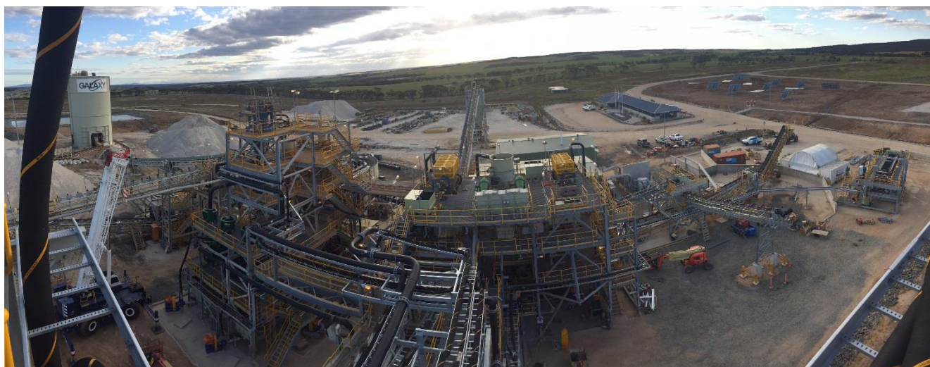
Mt Cattlin Nears Construction Completion
