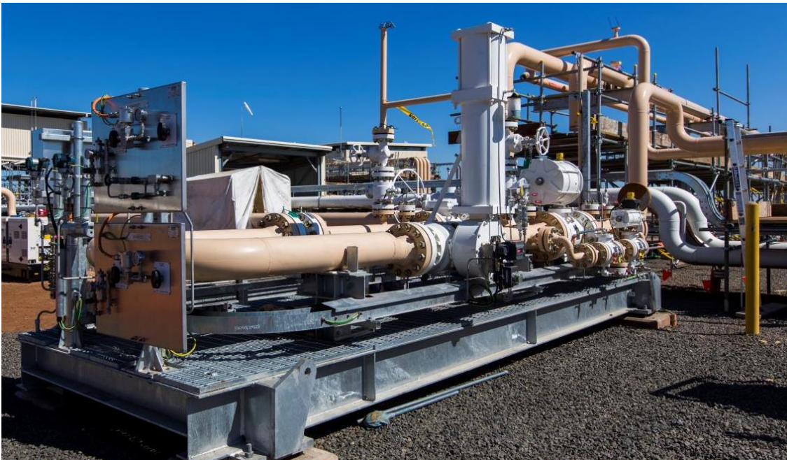
Flow reversal skid connects to pipeline for bi-directional flows
