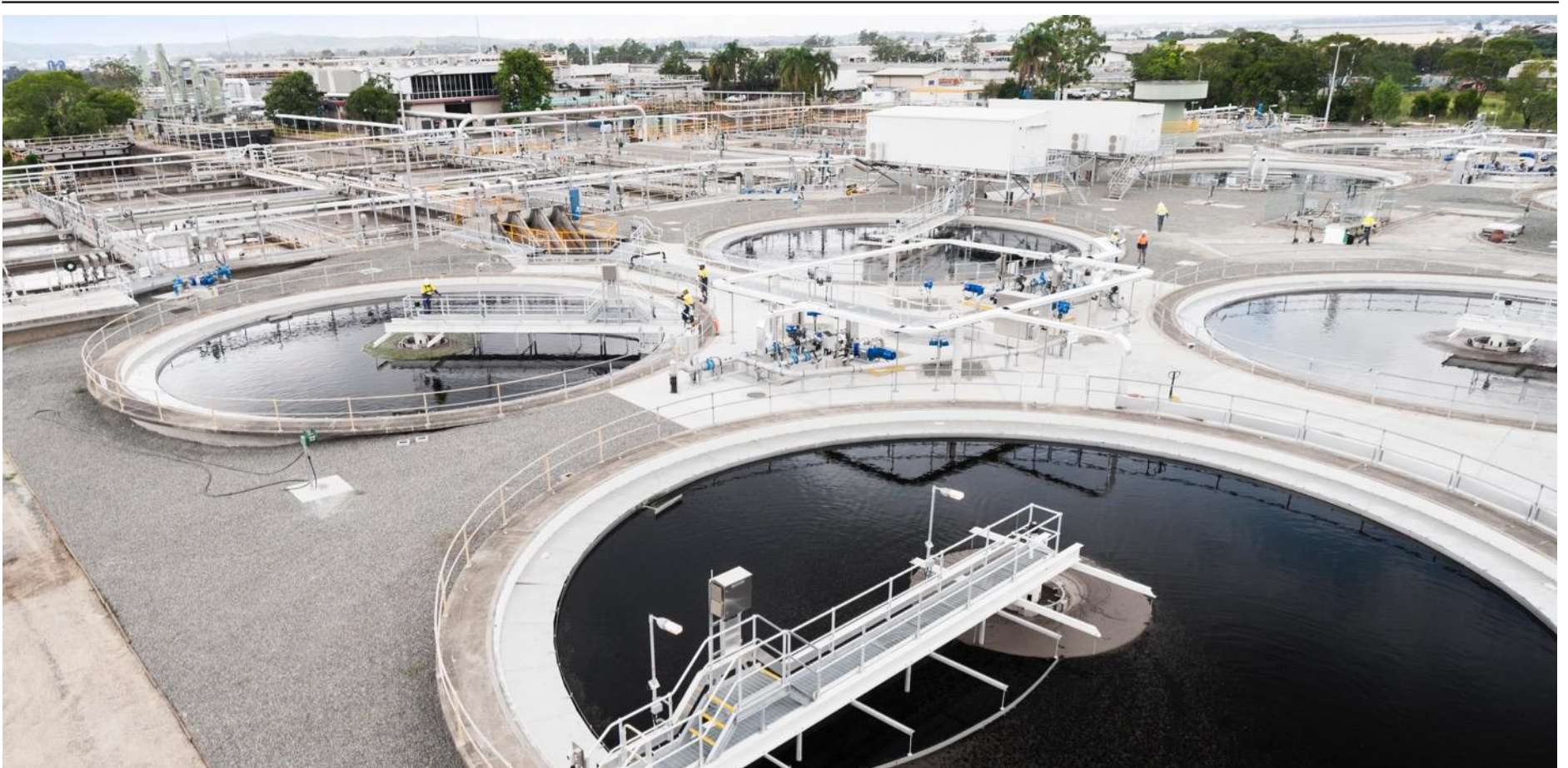
Oxley Creek Sewage Treatment Plant, Rocklea, Queensland
