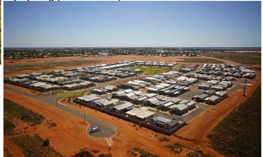
Osprey Village, South Hedland, Western Australia
