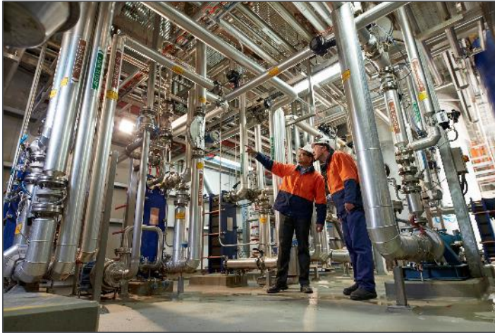
OILSEEDS CRUSHING/REFINING, NUMURKAH, VIC
