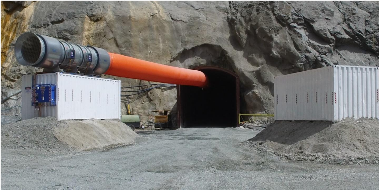
Figure 3: Syama Underground 1200 portal established
