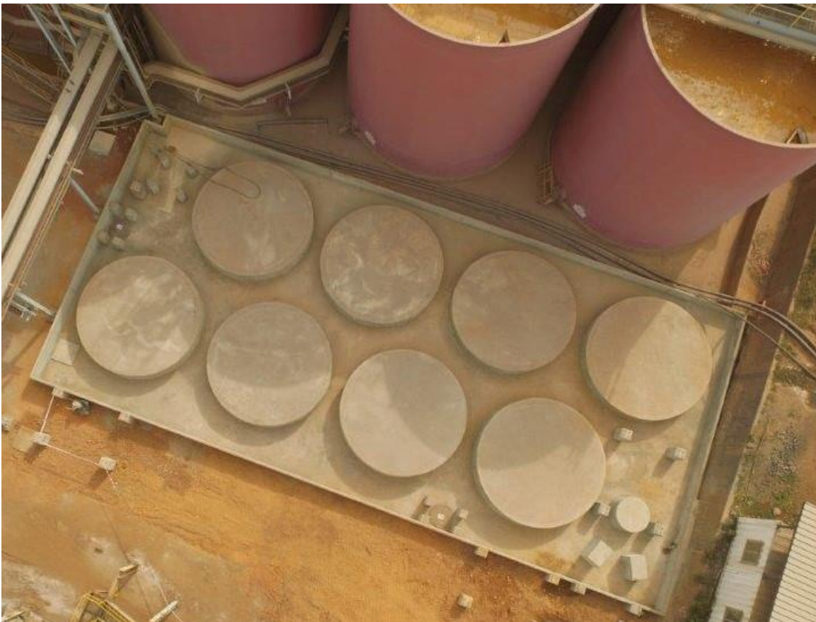
Figure 4: Syama Project 85 site civil work completed
