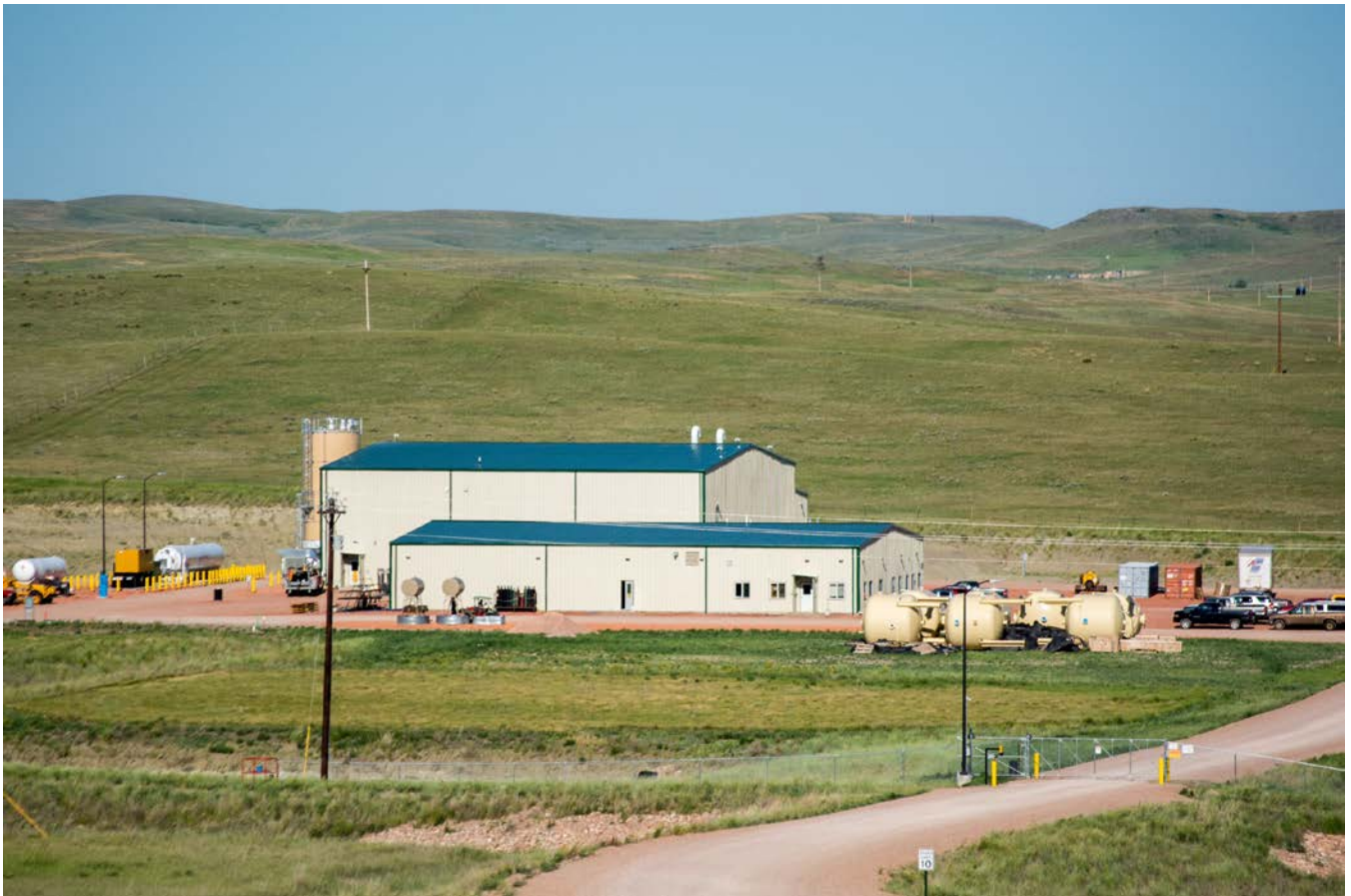
Figure 2: CPP and Admin Building, Lance Projects, Wyoming USA
