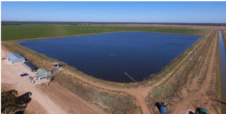
Water storage and pump station. Remaining capex will be applied to further irrigation infrastructure, water entitlements and planned initial maintenance costs. Image taken Dec 2016
