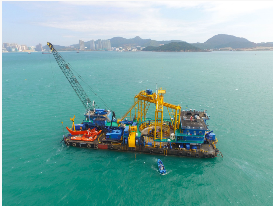
Challenger 8 Preparing to Install the TKO Express Cable
