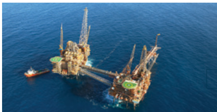
The Persephone Project is expected to supply gas to the North Rankin Complex from Q3 2017.
