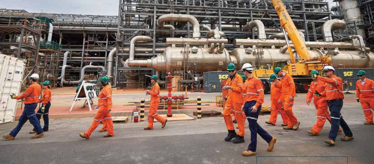
The Karratha Community Liaison Group completing a site tour as part of the planned turnaround activities at the Karratha Gas Plant.
