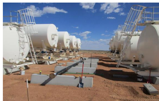
Bauer facility expansion.
