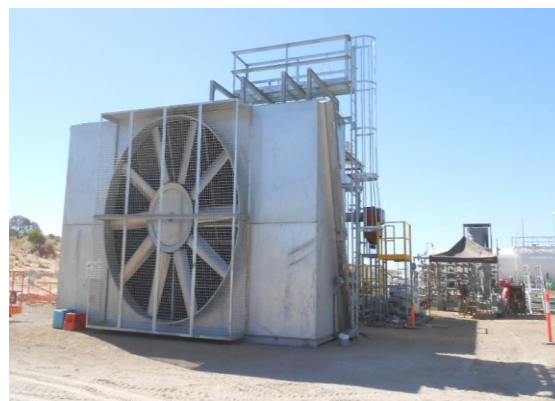
Installation of compression at Middleton.
