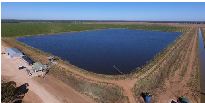
Water storage and pump station. Remaining capex will be applied to further irrigation infrastructure, water entitlements and planned initial maintenance costs. Image taken Dec 2016
