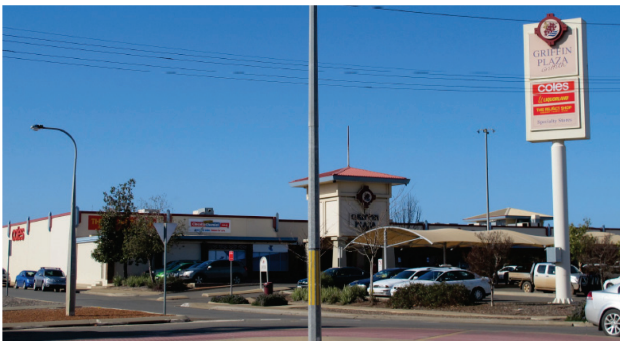
Griffin Plaza in Griffith NSW, will be the first centre to have Solar PV installed.
