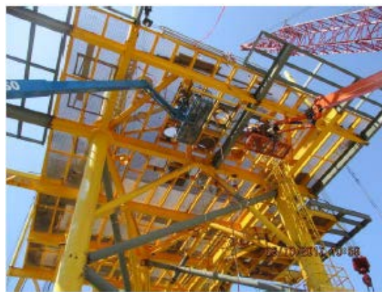
Decks under construction.
