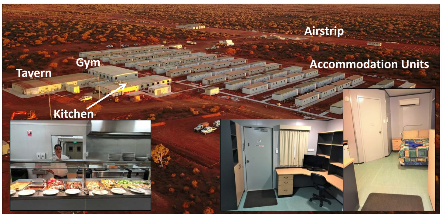
Photo 2: Dalgaranga Village Nearing Completion
