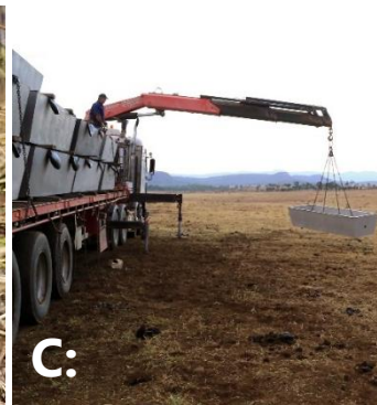
C: Installation of a water trough, June 2017
