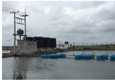
Power, storage silos, site office
