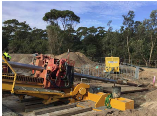
Horizontal directional drilling (HDD) in progress at Orbest
