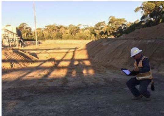
Bulk earthworks at Orbest
