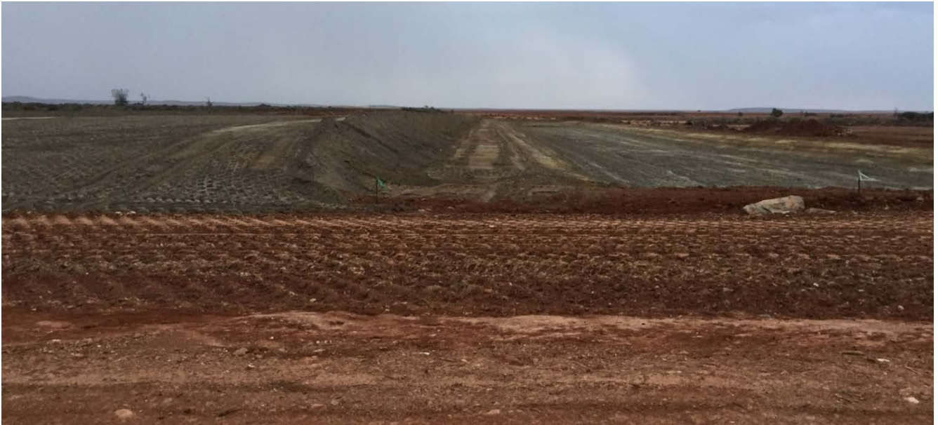
Photo 4: Dalgaranga Tailings Storage Facility Construction Progress
