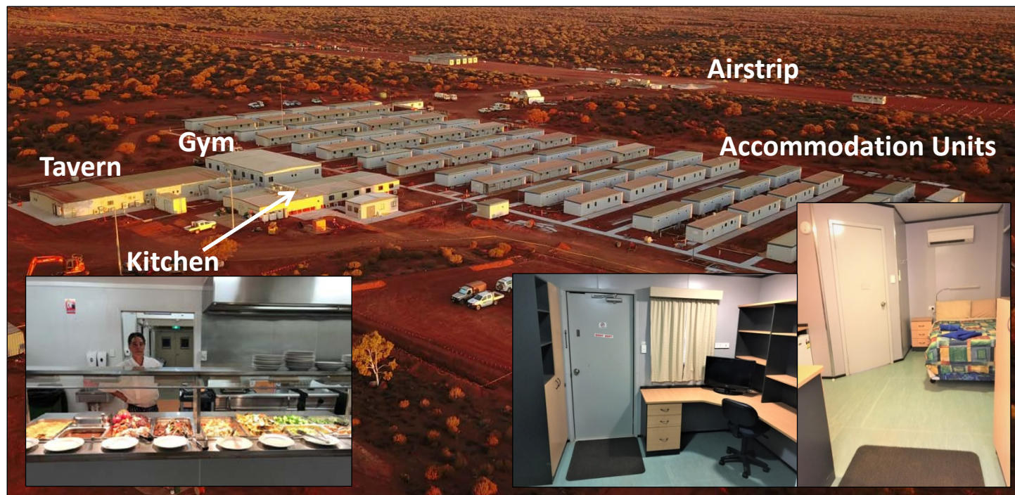
Photo 6: Dalgaranga Village Completed
