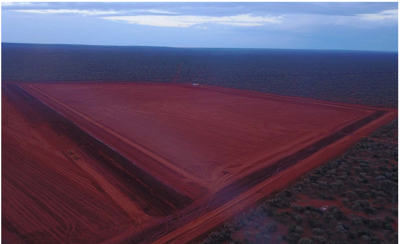
Photo 5: Dalgaranga Evaporation Pond Construction Progress
