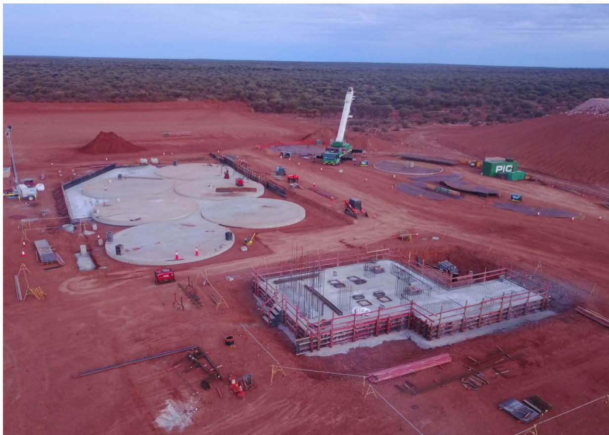
Photo 2: Dalgaranga Plant Site Concrete Progress
