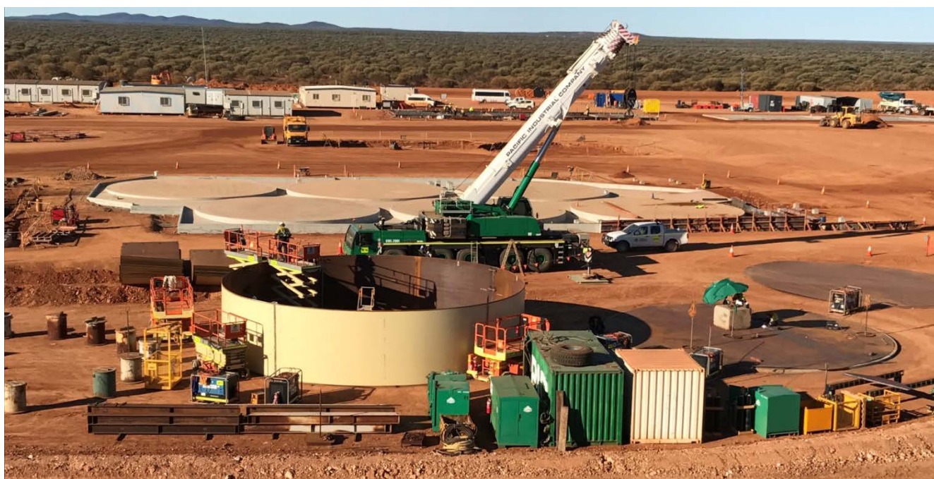
Photo 3: Dalgaranga Plant Site CIL Tank Construction Progress
