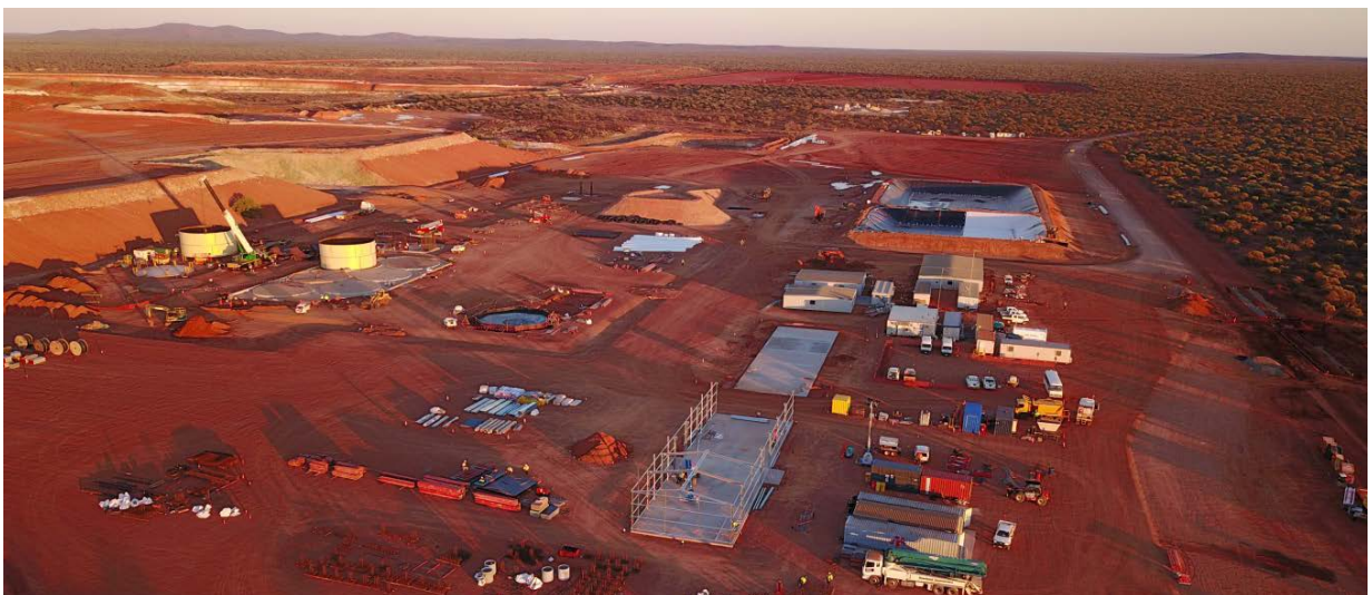
Construction of the Dalgaranga Gold Project Well Advanced
