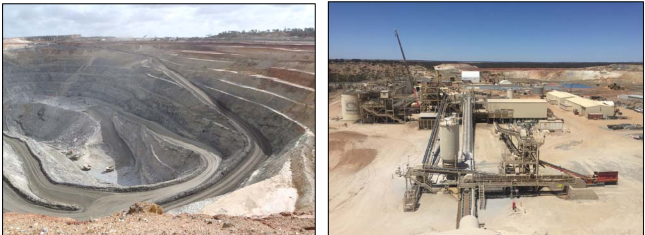
Figure 3: Edna May Stage 2 open pit (LHS) and processing plant (RHS)
