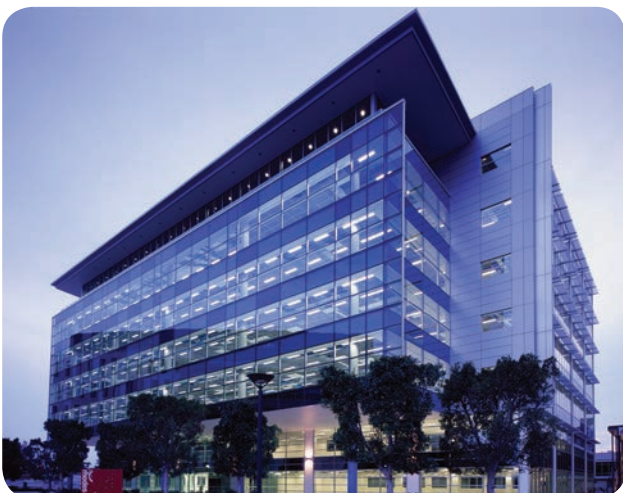
Building A, 1 Homebush Bay Drive, Rhodes
