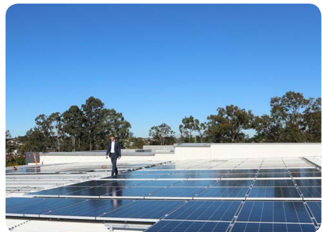
12 Electronics St – 100 Kilowatt installation being completed
