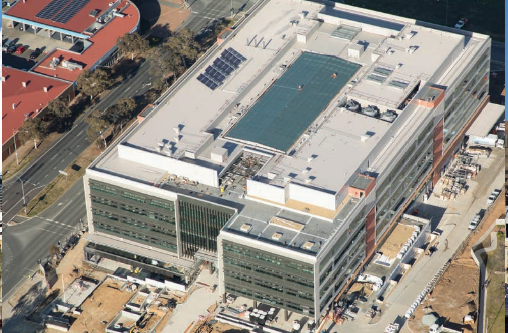
Tuggeranong Office Park, Greenway
