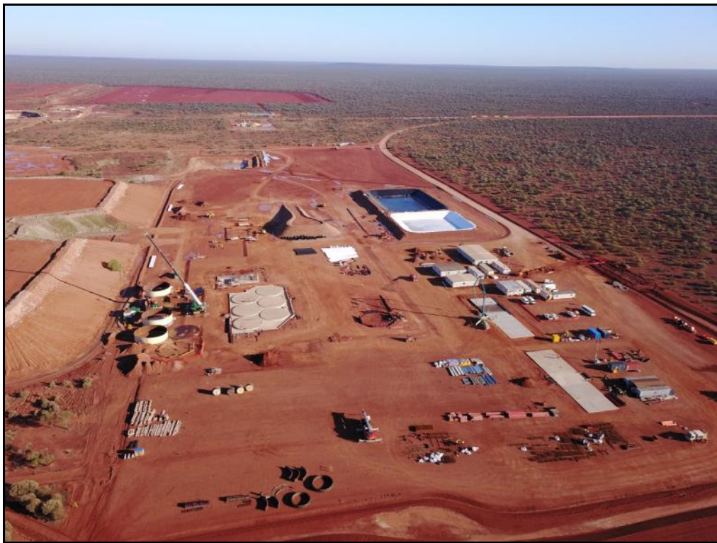
Photograph 3: 2.5Mtpa Processing Plant Site Construction Overview
