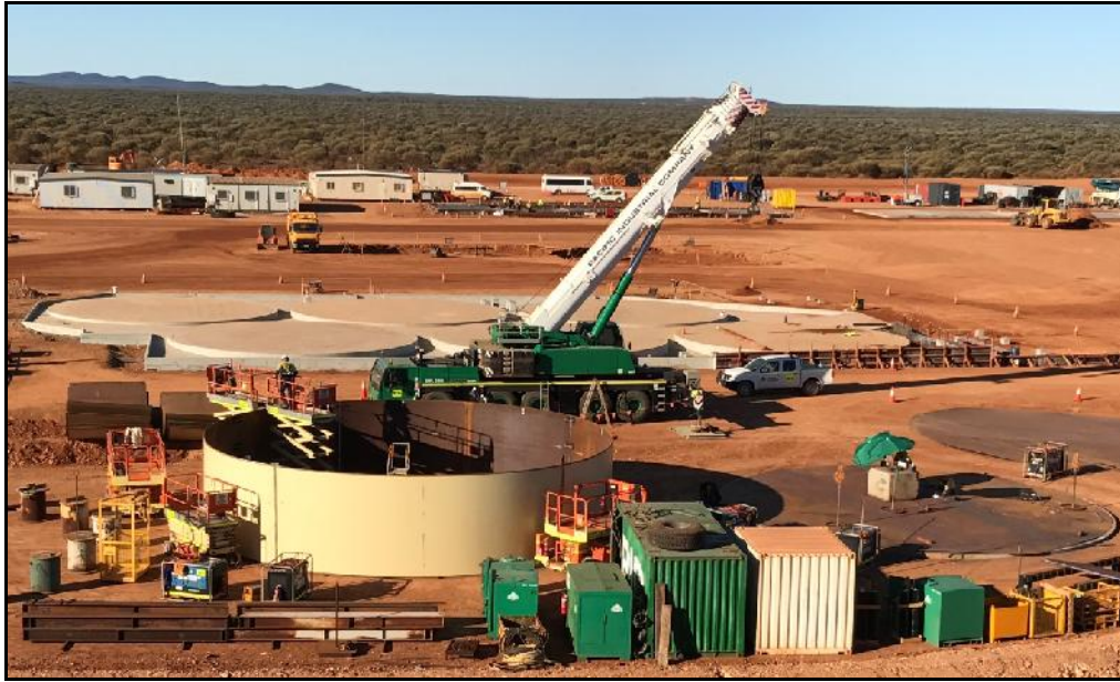
Photograph 2: CIL Tank Construction Underway
