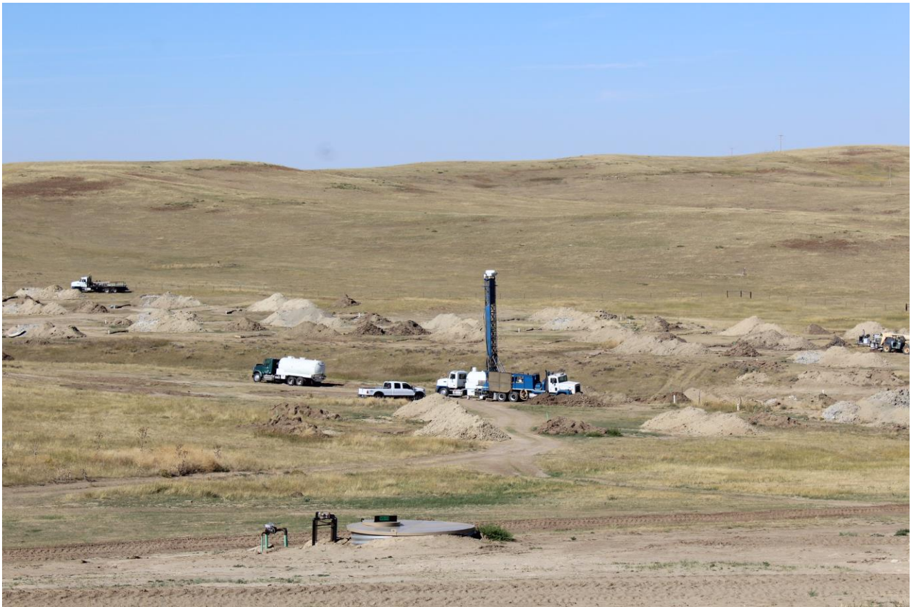
Figure 5: Drill Rig, Header House 10, Lance Projects, Wyoming USA
