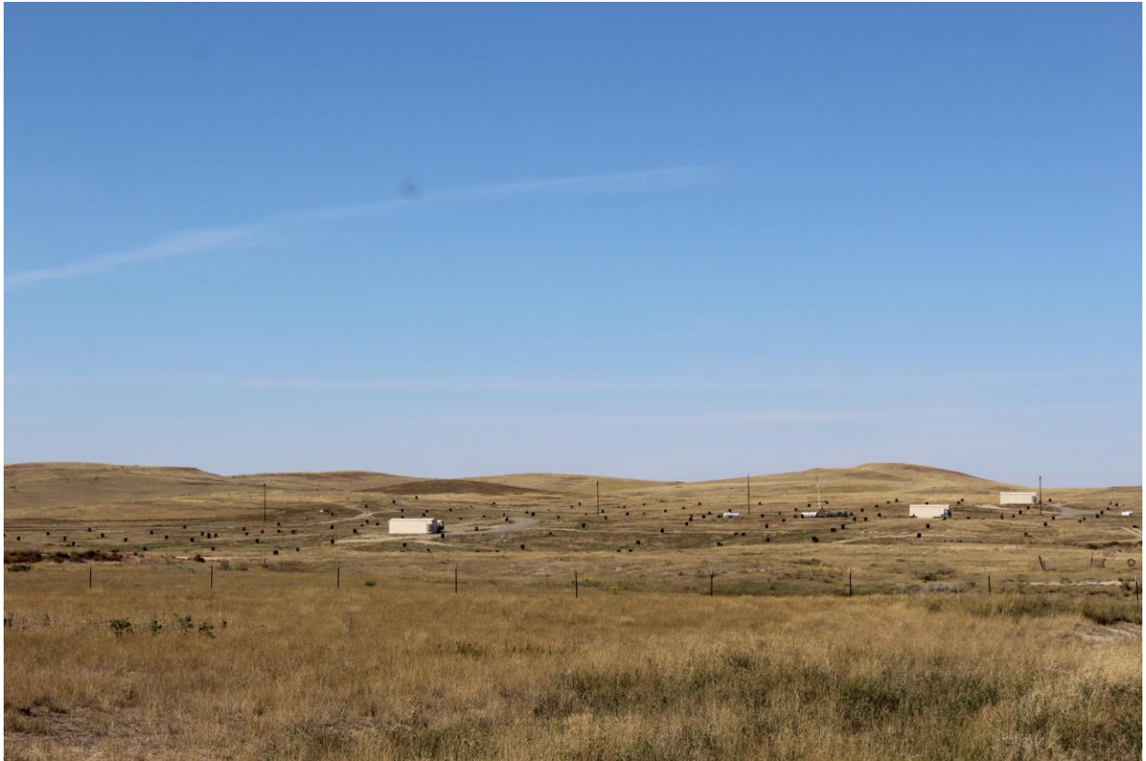
Figure 3: Wellfield and Header Houses, Mine Unit 1, Lance Projects, Wyoming
