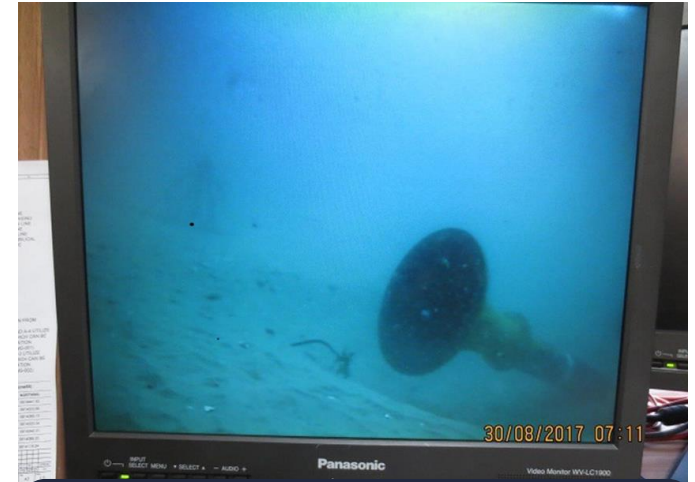
Umbilical bell mouth completed & ready
