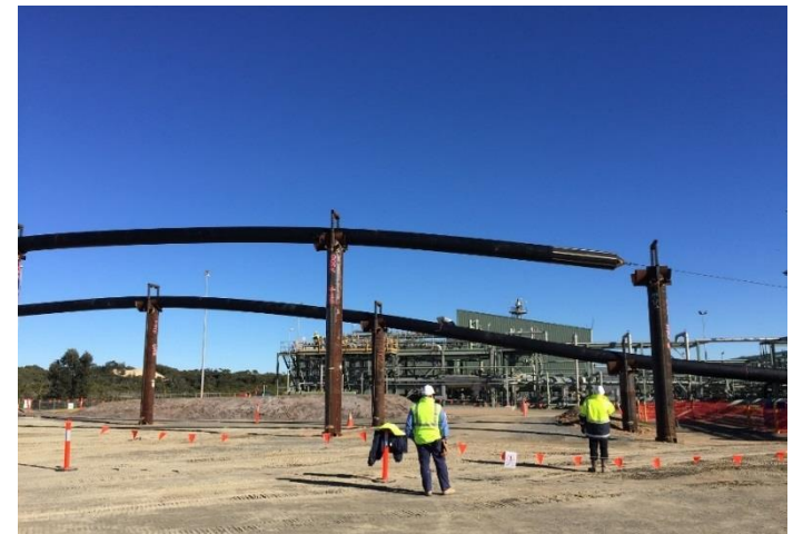
Casing pull-through to HDD
