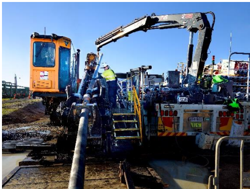
Horizontal directional drill (HDD) of shore crossing
