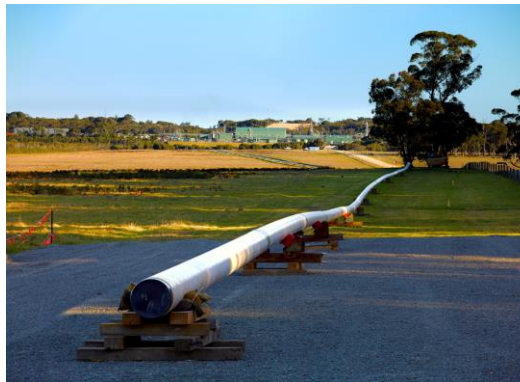
Welded shore crossing pipe, laid out to plant ready to be pushed through HDD
