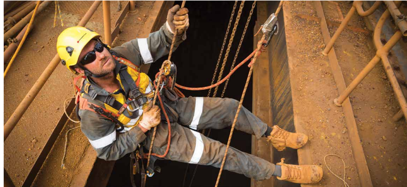
IMAGE A member of the Monadelphous rope access team entering a train loadout bin for inspection at BHP's Mining Area C, Newman, Western Australia.
