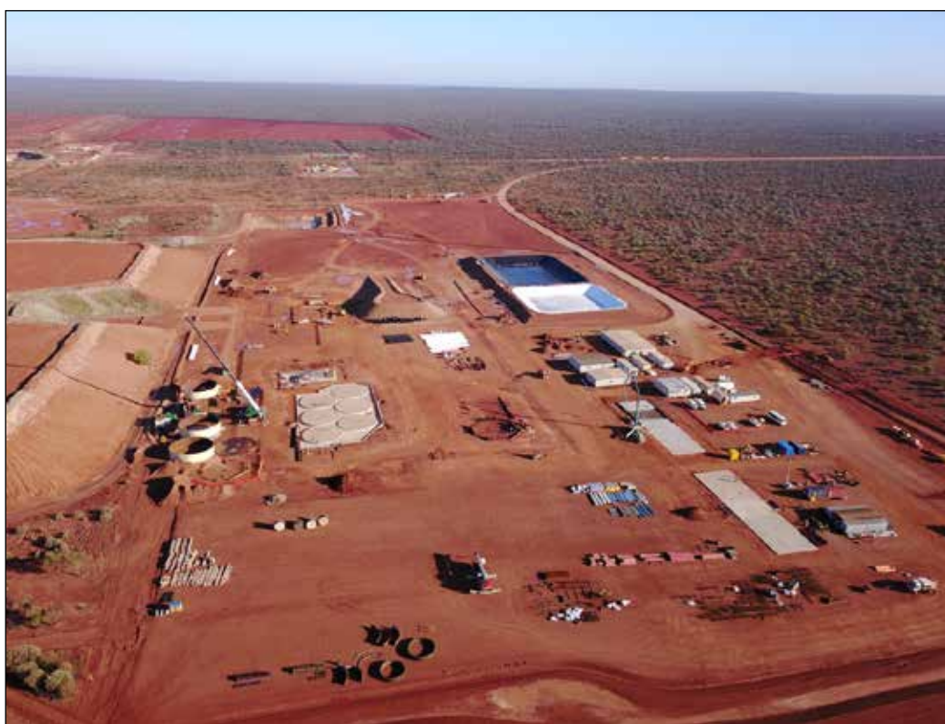
Photograph 3: 2.5Mtpa Processing Plant Site Construction Overview
