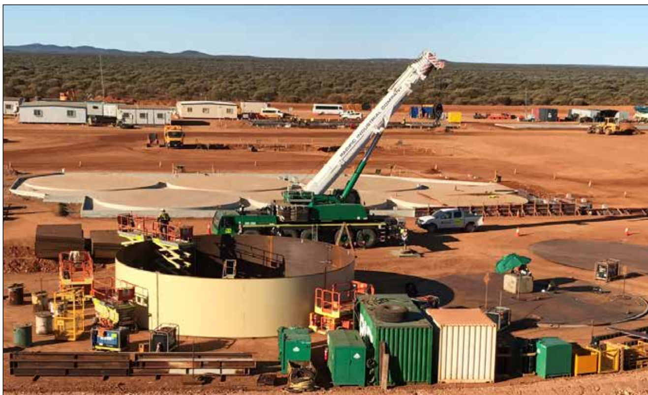
Photograph 2: CIL Tank Construction Underway
