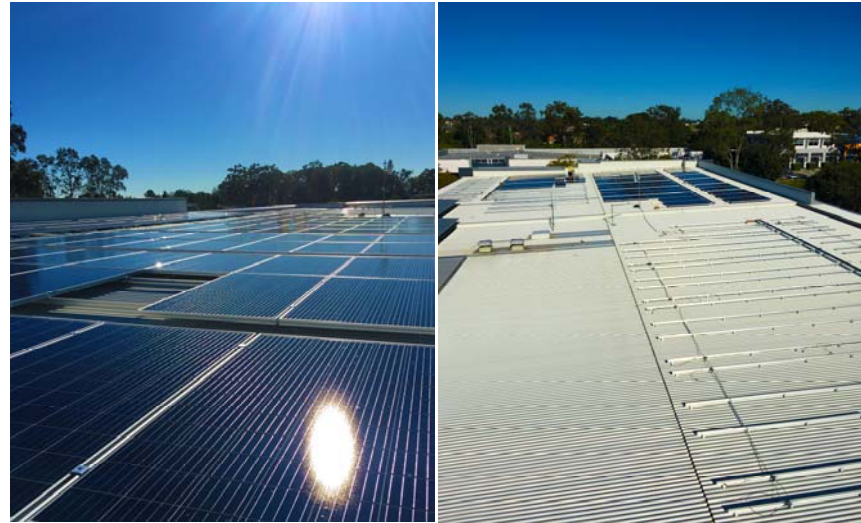
12 Electronics St – 100 Kilowatt installation being completed
