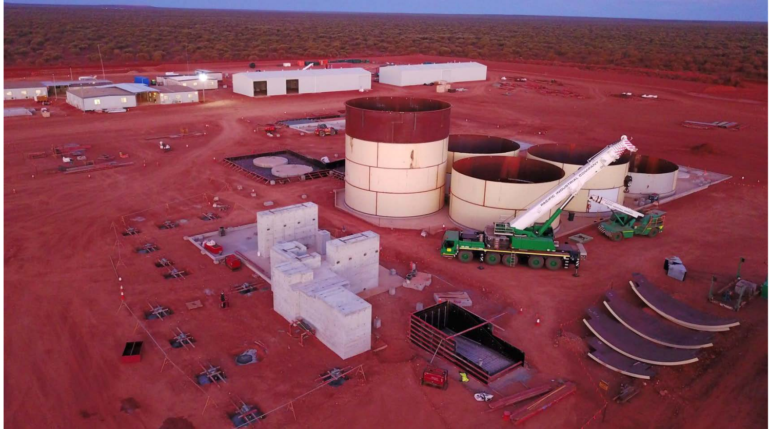
SAG Mill Foundations and CIL Tanks
