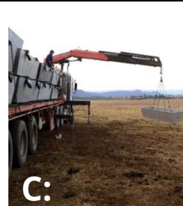
Installation of a water trough, June 2017
