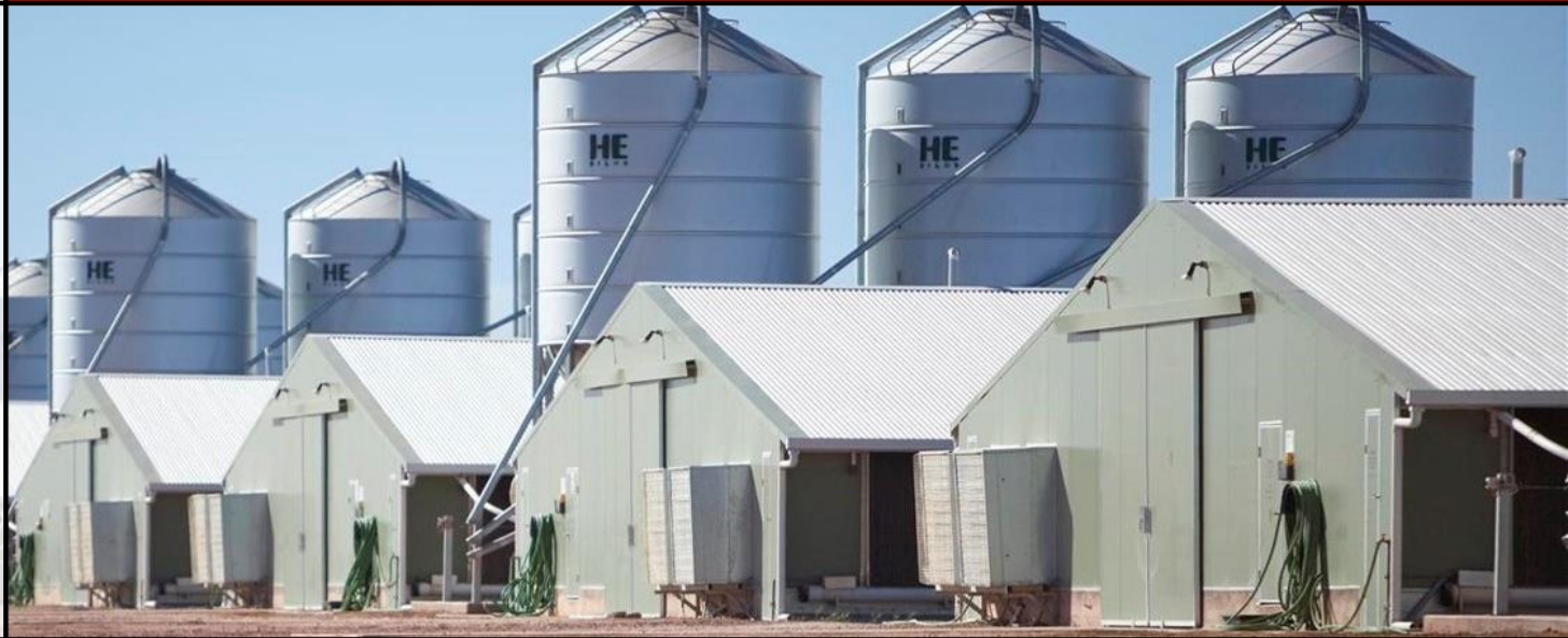
Griffith Poultry sheds, NSW 2009
