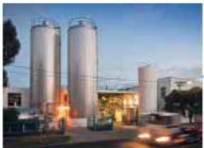
COBURG 10-16 Allenby Street Coburg VIC 3058 Australia
