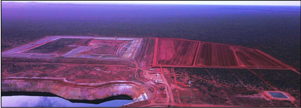
Photo 4: Evaporation Pond construction Complete (RHS) and TSF Lift Underway (LHS)
