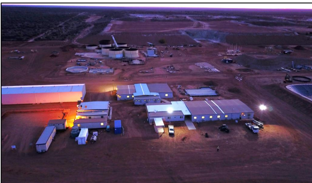
Photo 2: Associated Plant Site Infrastructure including Office Complex, Workshop and Warehouse
