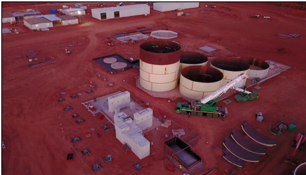
Photo 1: Construction of the SAG Mill Foundations and Leach Tanks Well Advanced
