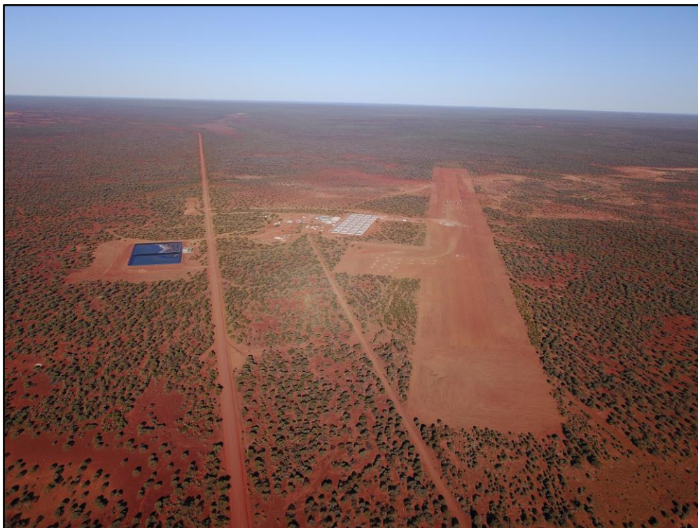
Photo 3: Airstrip Clearing Completed in Preparation for Runway Construction
