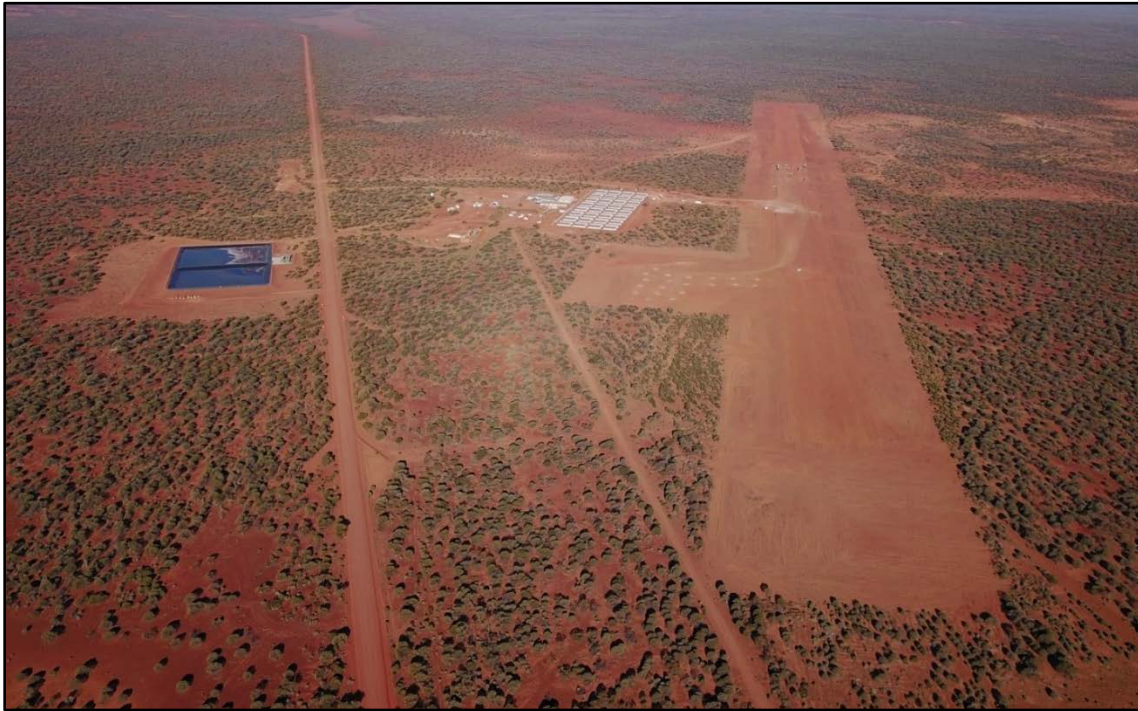
Photo 9: Dalgara Airstrip clearing
