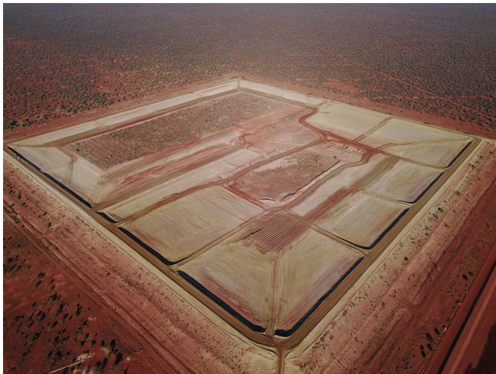
Photo 6: Dalgaranga Tailings Storage Facility Construction Progress
