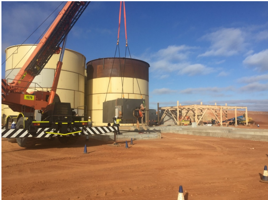
Photo 4: Installation of the Mechanical Equipment has commenced - Elution Heater being installed
