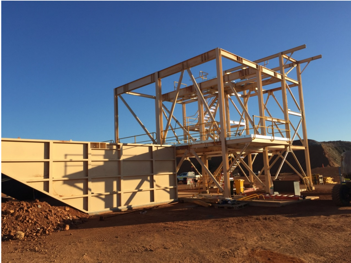
Photo 3: Steel Erection around the Transfer Bin
