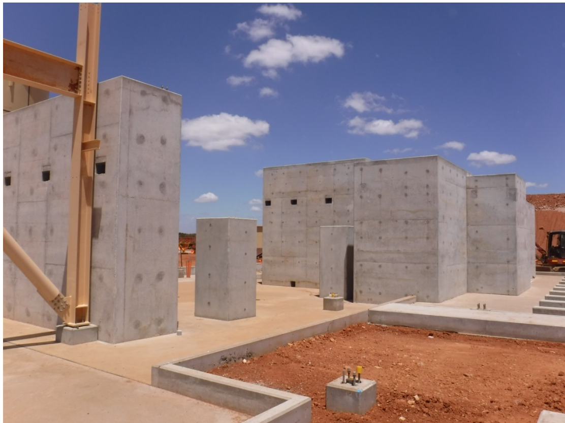
Photo 2: SAG Mill Foundations Completed
