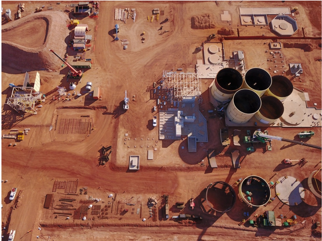
Photo 1: Dalgaranga Plant Site Construction Progress
