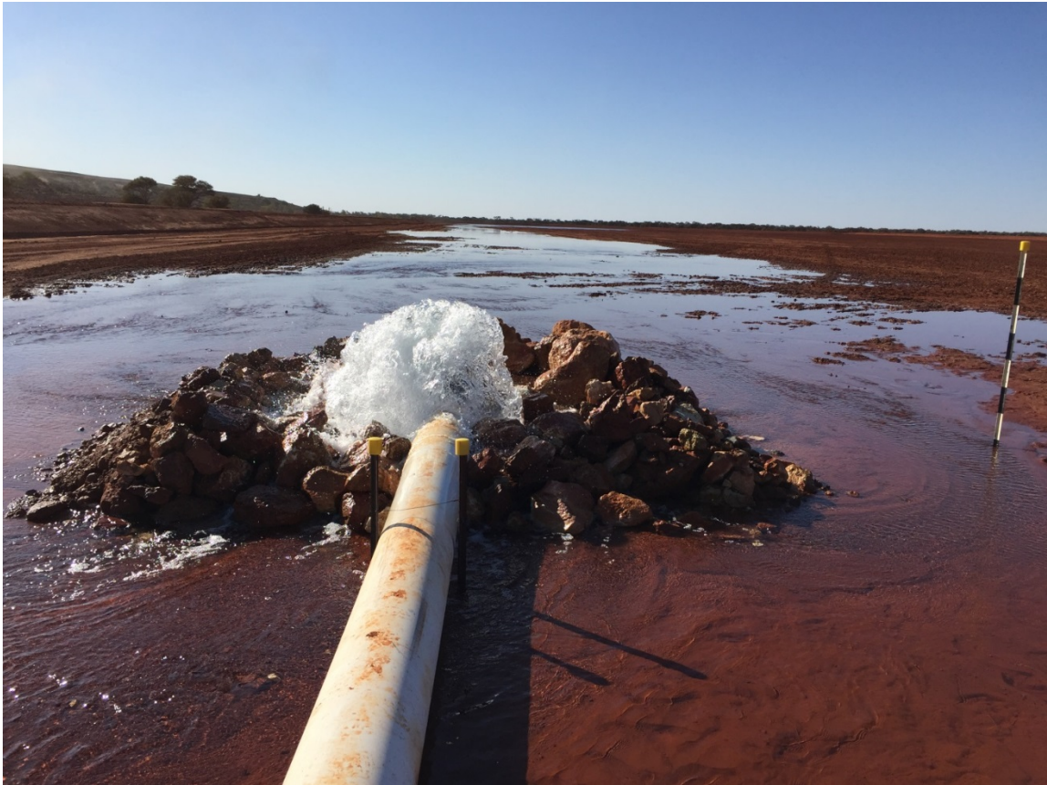
Photo 7: Gilbeys Dewatering Underway
