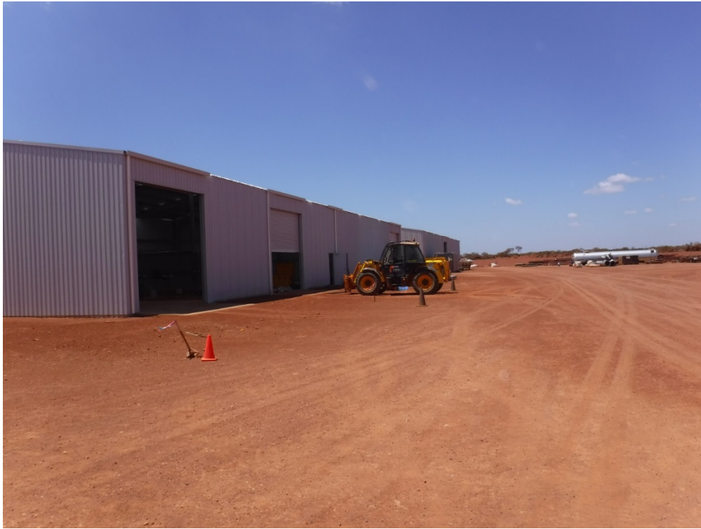
Photo 5: Workshop and Warehouse Construction Complete
