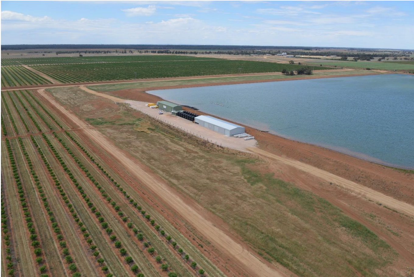
Pump station, fertigation system and 800 ML water storage cell to support 2016 plantings. Kerarbury, NSW, October 2017
