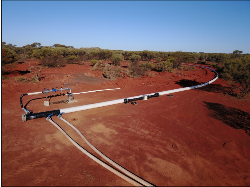
Dewatering Bores Completed and Pumping Underway
