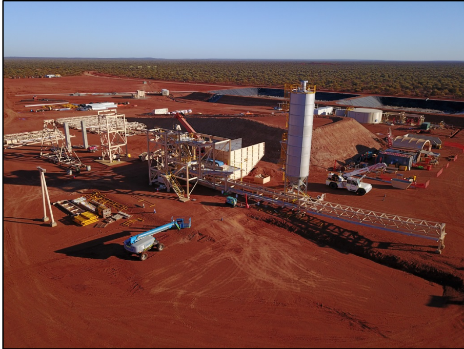
Transfer Bin & Lime Silo Construction
