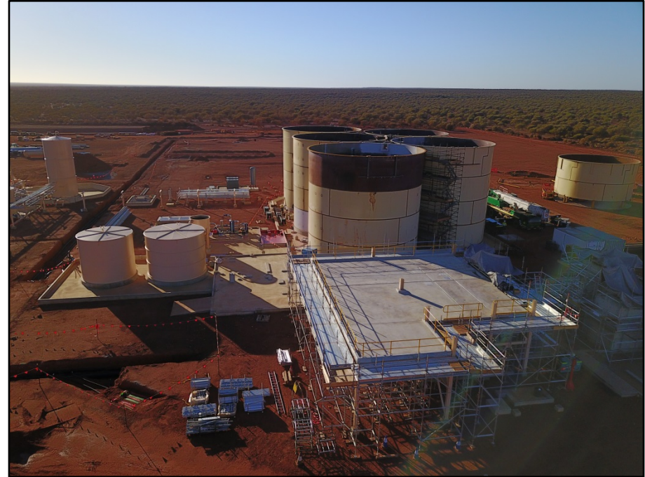
CIL Tanks & Milling Area
