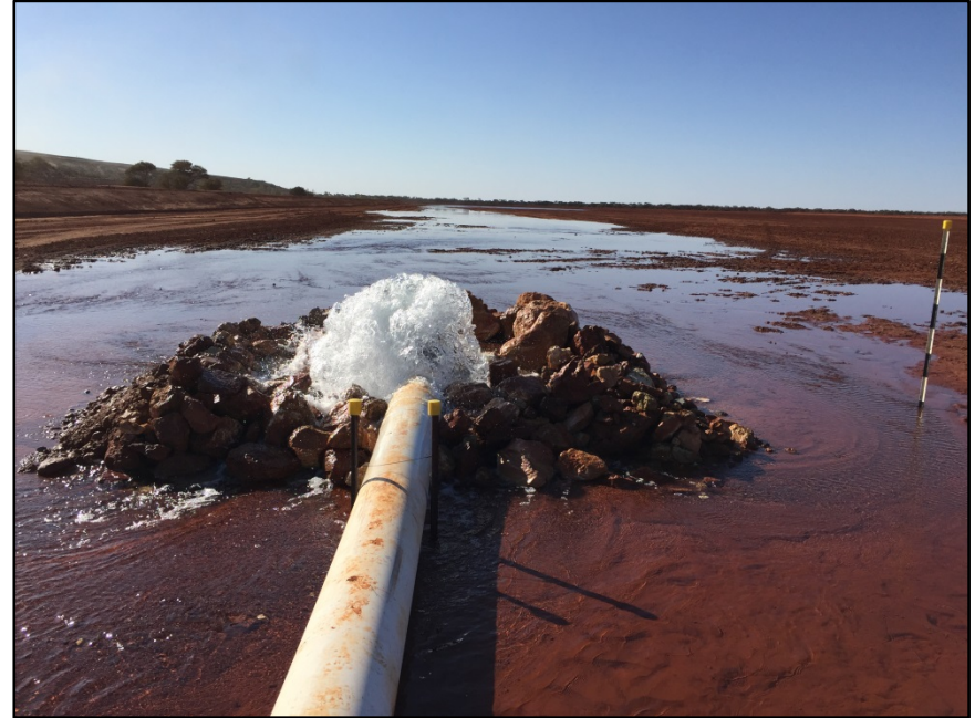
Evaporation Pond Completed and in Use
