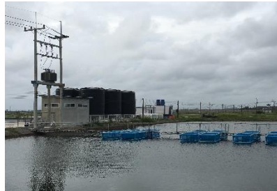
Power, storage silos, site office
