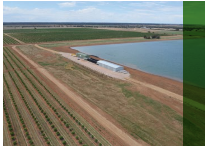
Pump station, fertigation system and 800 ML water storage cell to support 2016 plantings. Kerarbury, NSW, October 2017
