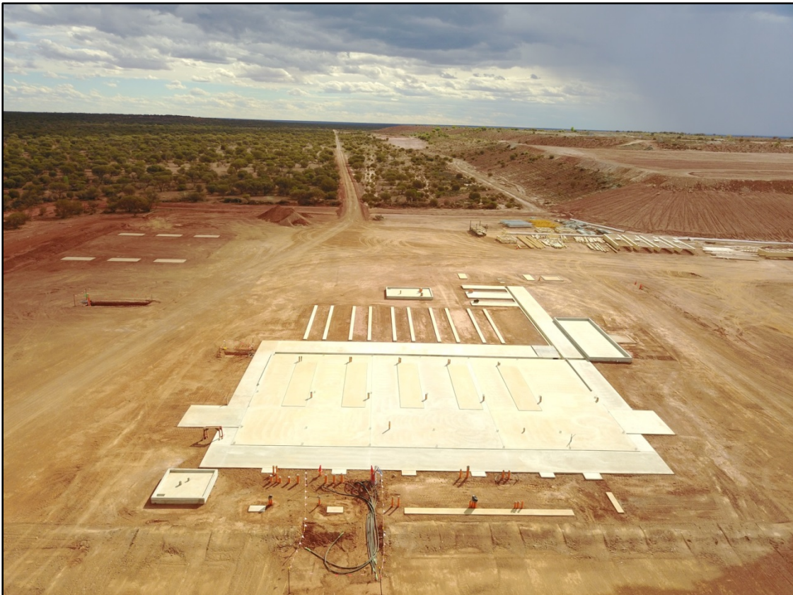
Photo 10: Power Station and Fuel Storage Foundations Complete
