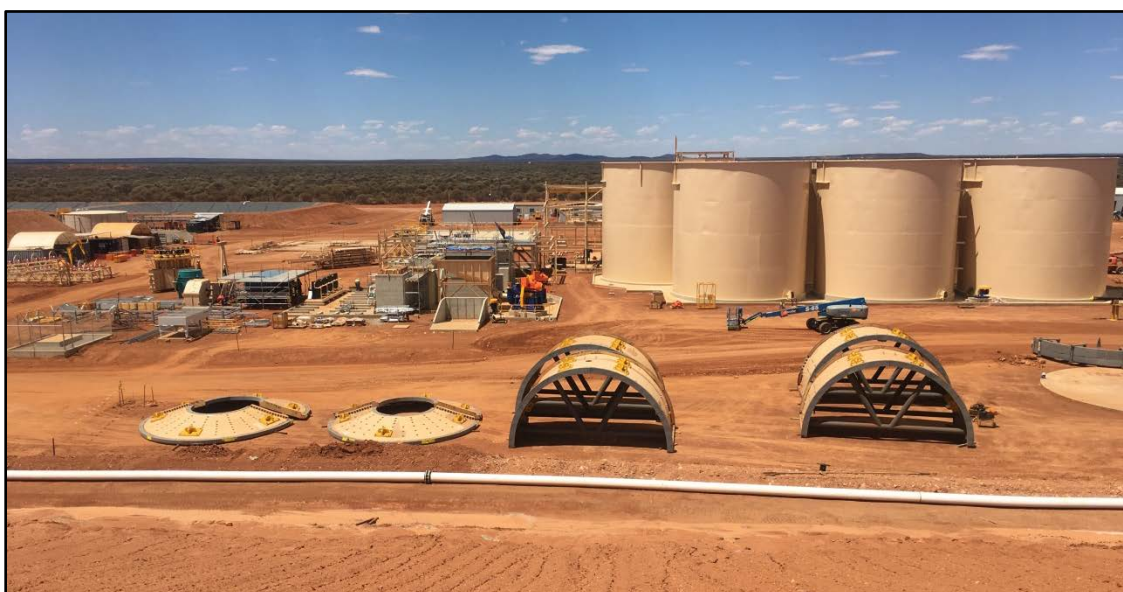
Photo 6: SAG Mill Shell and Mill Ends Onsite with Mill Foundations with CIL Tanks in the Background
