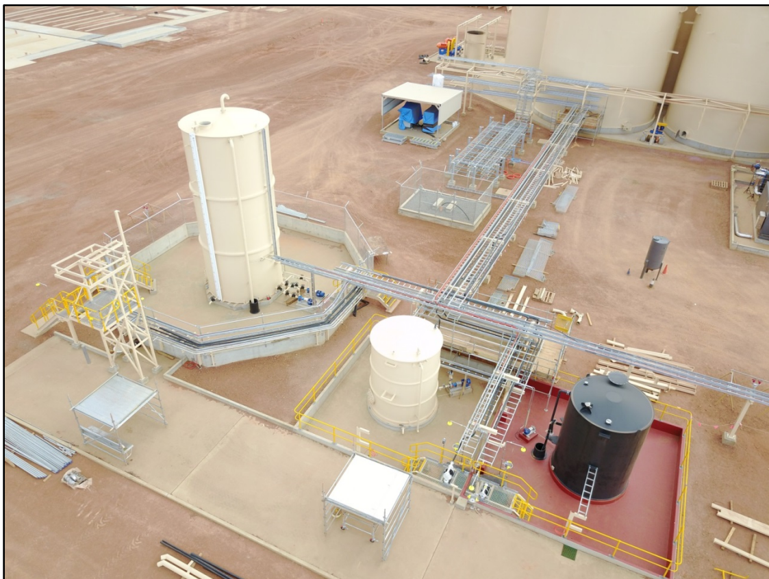
Photo 8: Reagent Storage Area - Nearing Completion
