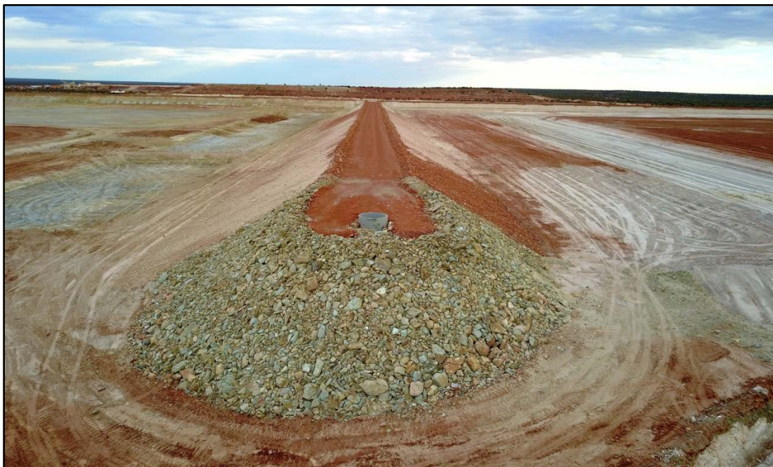
Photo 12: Dalgaranga TSF Decant Structure
