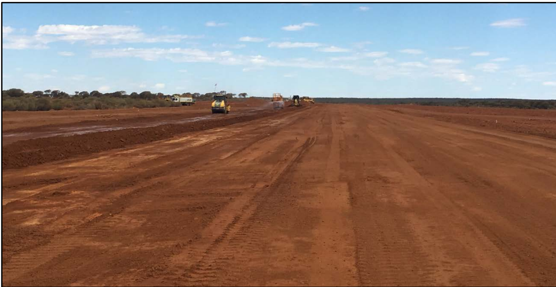
Photo 14: Dalgara Airstrip Construction Well Advanced
