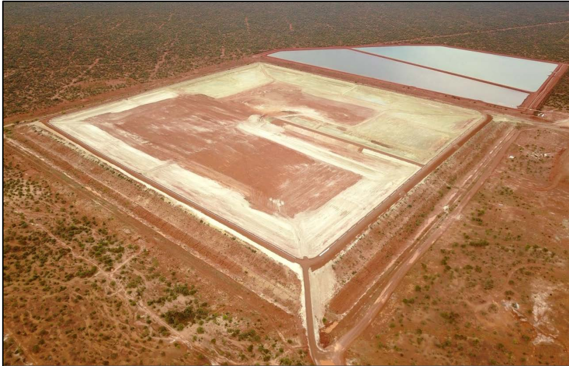
Photo 11: Dalgaranga Tailings Storage Facility (foreground) and Evaporation Ponds In Use (background)
