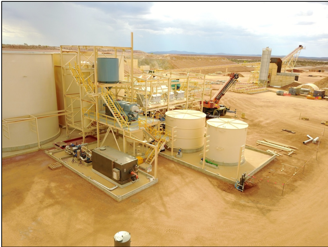
Photo 7: Elution and Gold Recovery Circuit Construction and Installation Well Advanced
