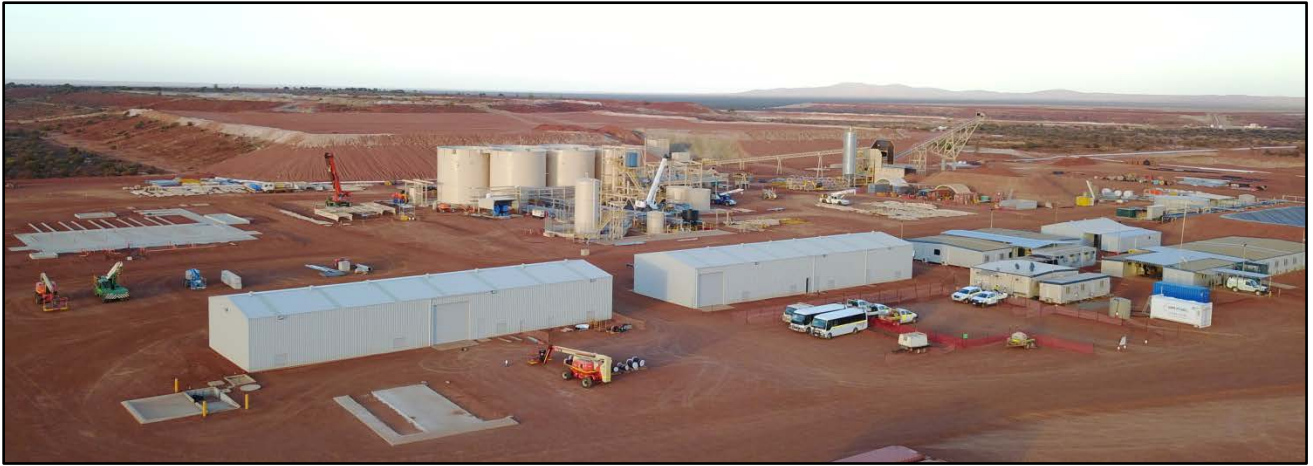
Photo 1: Dalgarranga Plant Site Construction Progress
