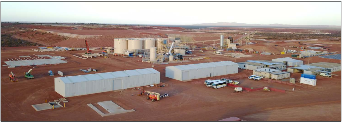
Photo 1: Dalgaranga Plant Site Construction Progress
