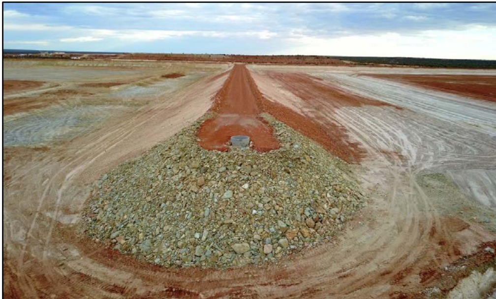
Photo 12: Dagaranga TSF Decant Structure
