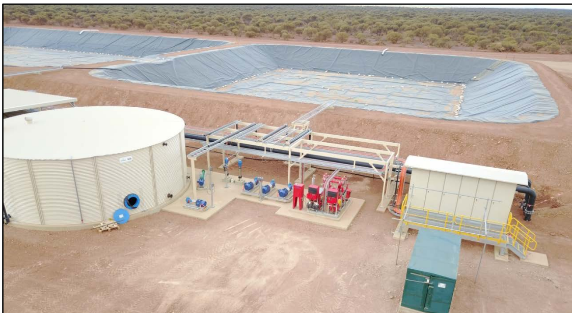
Photo 9: Water Services Area - Well Advanced
