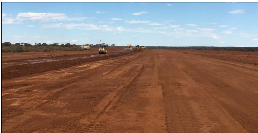
Photo 14: Dagaranga Airstrip Construction Well Advanced
