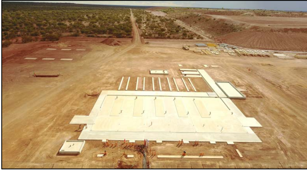
Photo 10: Power Station and Fuel Storage Foundations Complete
