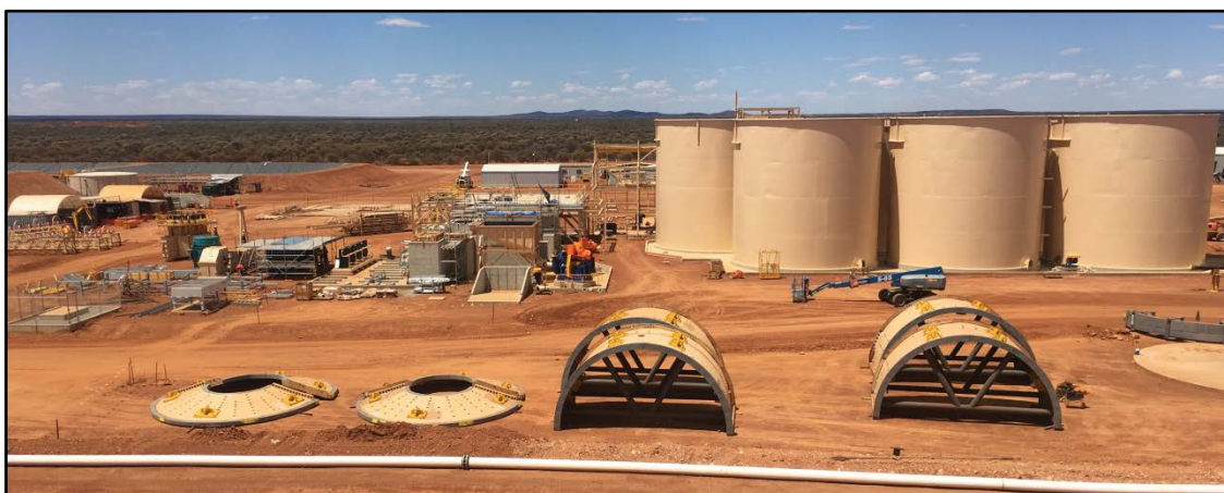
Photo 6: SAG Mill Shell and Mill Ends Onsite with Mill Foundations with CIL Tanks in the Background
