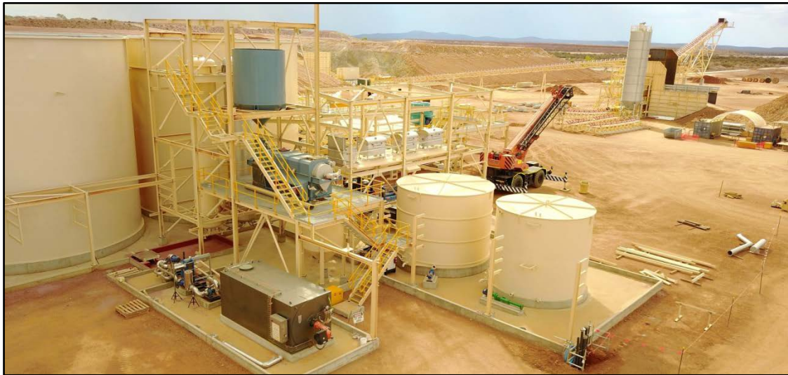
Photo 7: Elution and Gold Recovery Circuit Construction and Installation Well Advanced
