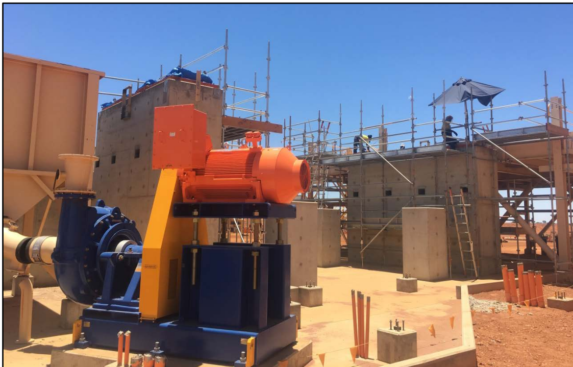
Photo 5: SAG Mill Foundations and Main Cyclone Feed Pumps
