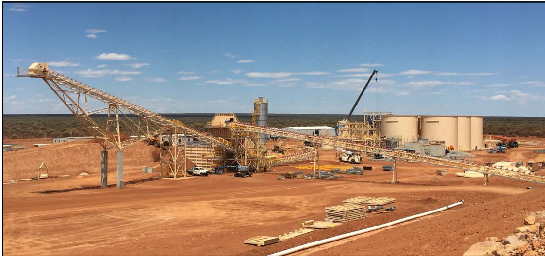
Photo 4: Ore Stockpile Conveyor (CIL Tanks and SAG Mill Foundations in background)
