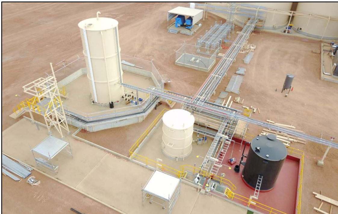
Photo 8: Reagent Storage Area - Nearing Completion
