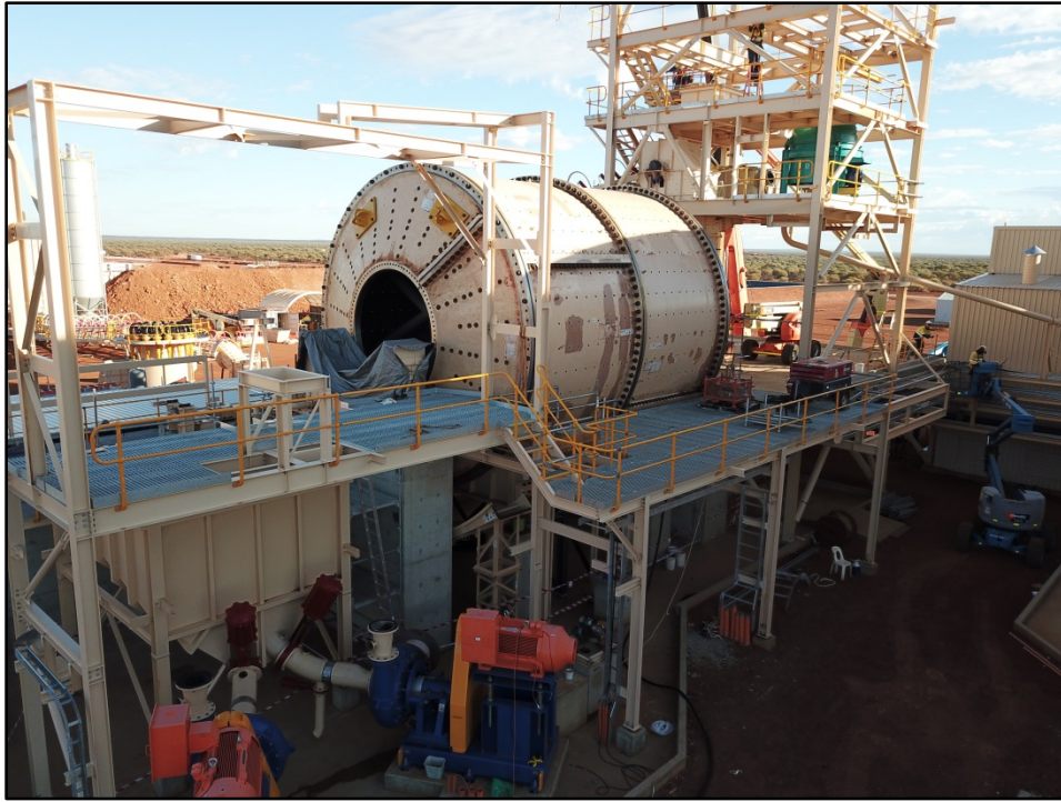
Photo 3: SAG Mill Installation – Progressing Well
