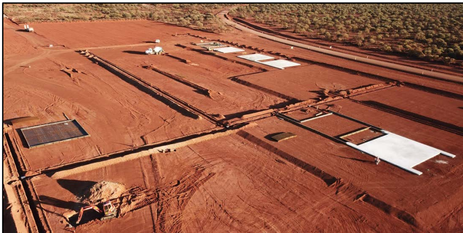
Photo 8: NRW Site Establishment Underway Including Maintenance Workshops, Offices and Associated Infrastructure
