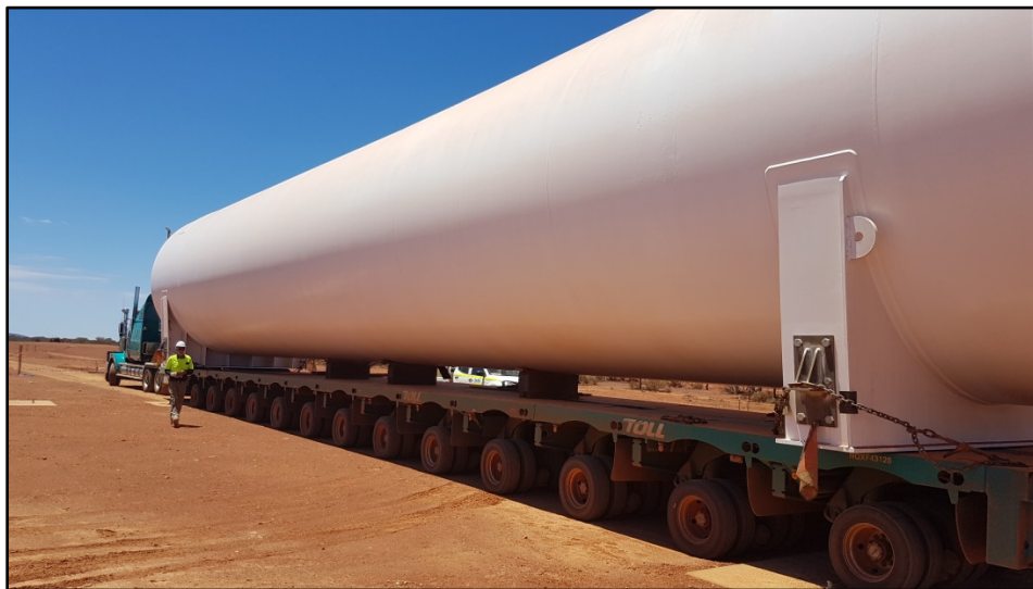
Photo 7: EVOL's LNG Fuel Storage Tank Being Delivered to Site
