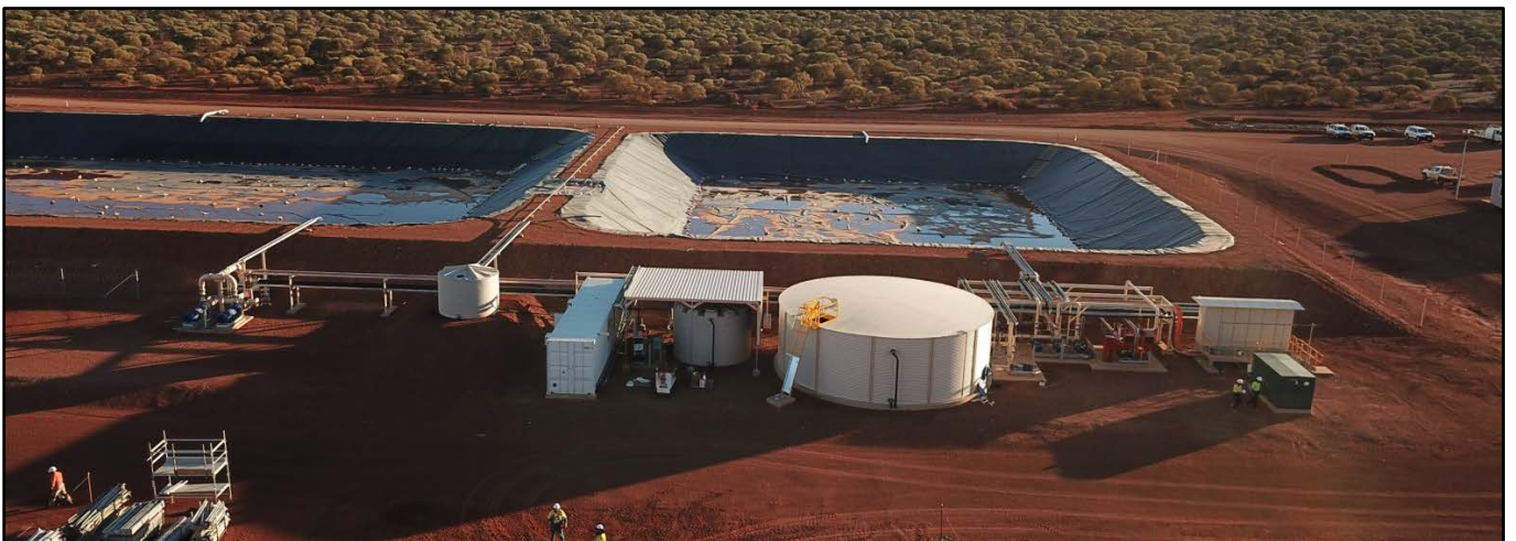
Photo 5: Water Services Area – Ready for Commissioning
