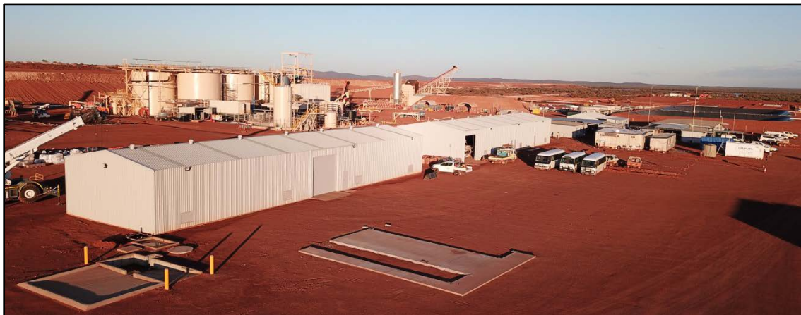
Photo 1: Dalgaranga Plant Site Construction Progress
