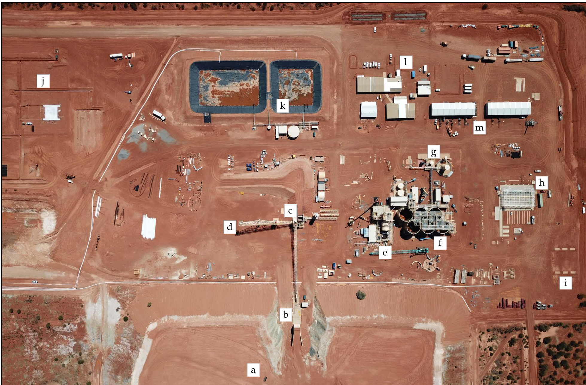
Photo 2: Dalgaranga Process Plant Site Overview
