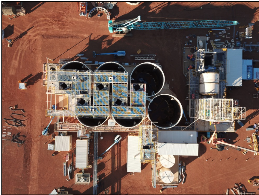
Photo 4: Top of CIL Tank Steelwork, SAG Mill and Cyclone Tower Construction - Well Advanced
