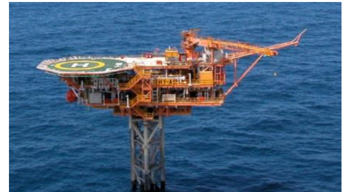
Thylacine well head platform
