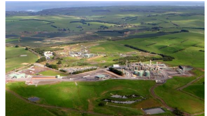
Otway gas plant
