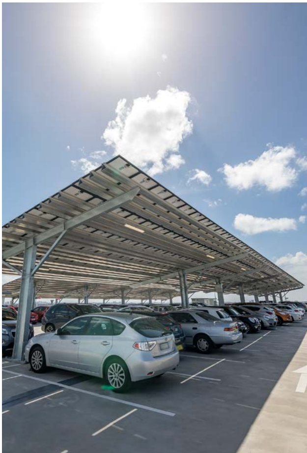
New solar installation on top of the P6 car park at T1 International.
