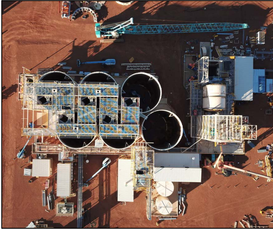
Top of CIL Tank Steelwork, SAG Mill and Cyclone Tower
