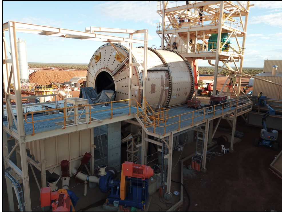
SAG Mill Installation
