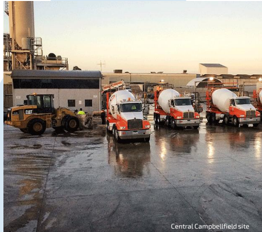
Central Campbellfield site
