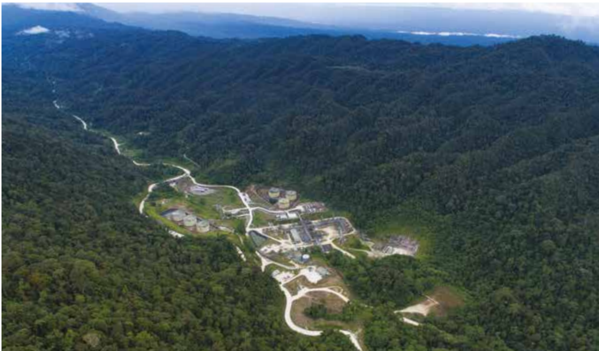
Oil Search's Central Processing Facility, located in the Southern Highlands of PNG, underwent a 17 day scheduled maintenance outage in 2017, to help ensure ongoing safe and reliable operations.
